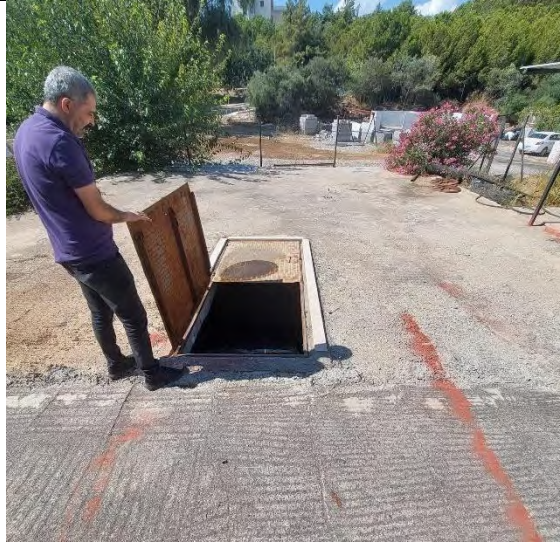
Rainwater Harvesting System - Cistern (water reservoir)
