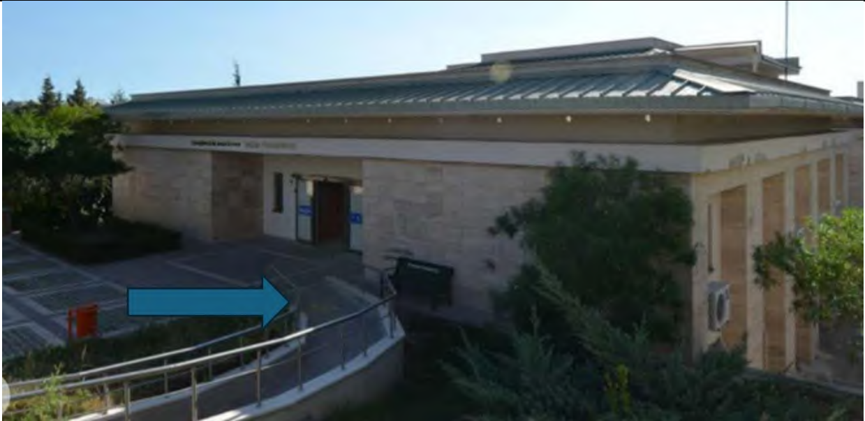
Mersin University disabled ramp
