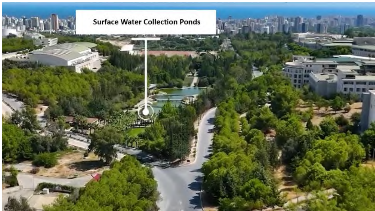
Surface Water Collection Ponds
