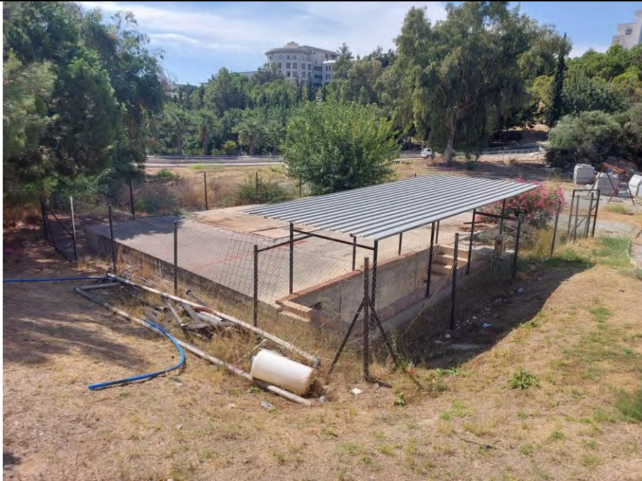
Rainwater Harvesting System
