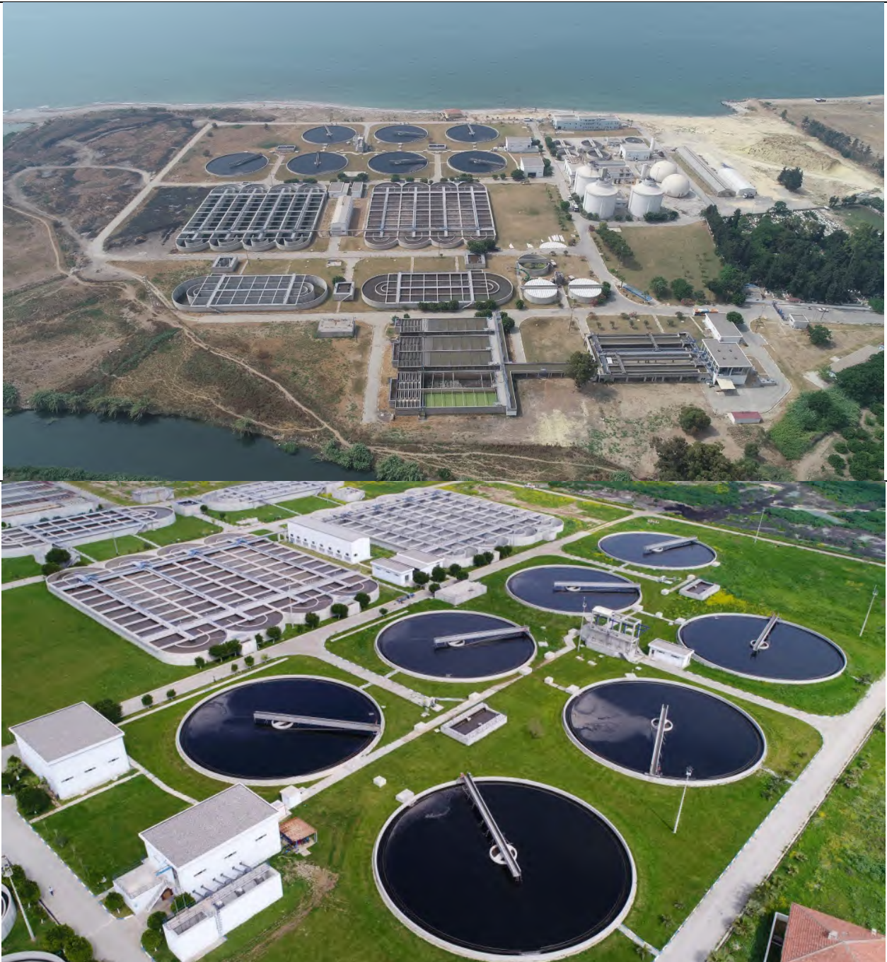
Karaduvar Wastewater Treatment Sytem (Mersin, Turkey)
