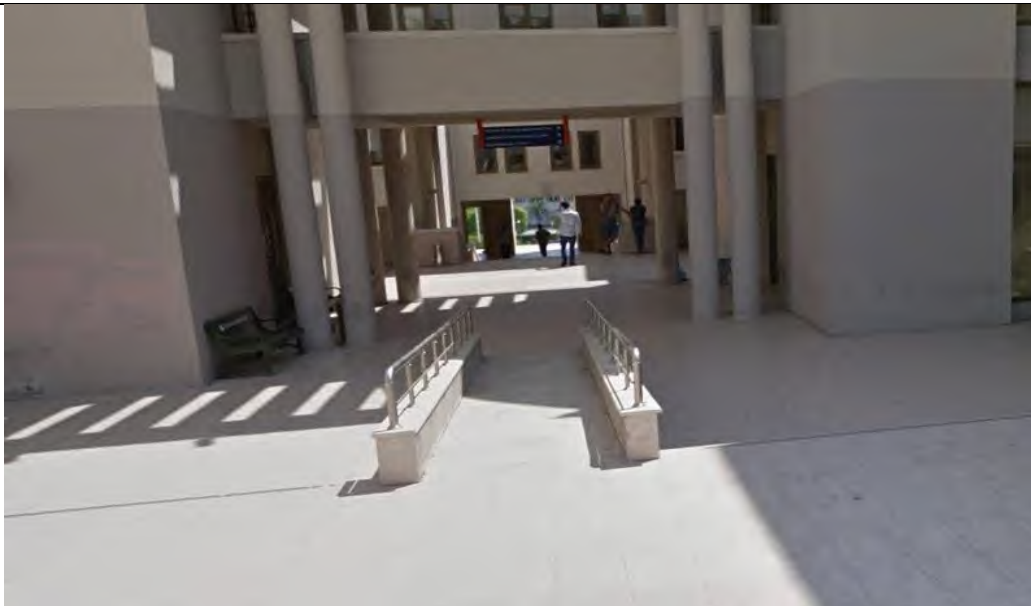
Mersin University disabled ramp
