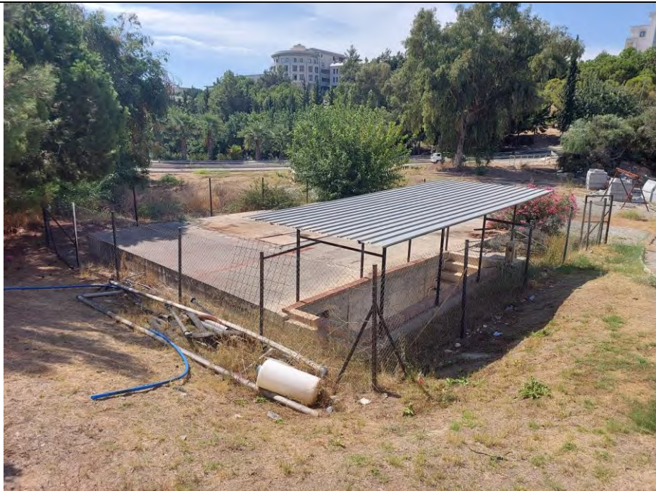
Rainwater Harvesting System
