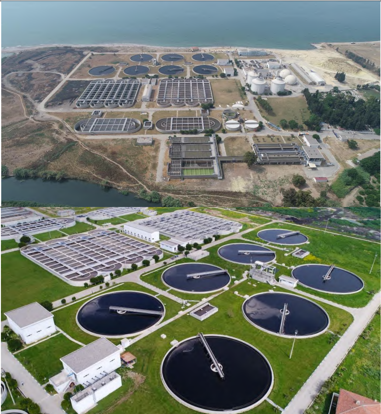
Karaduvar Wastewater Treatment Sytem (Mersin, Turkey)
