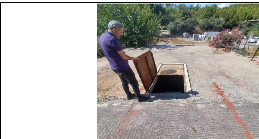
water booster for irrigation - Cistern (In Ground Water Tank)
