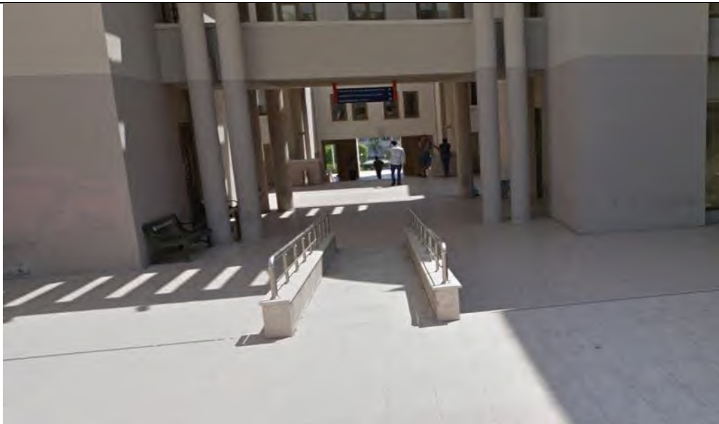
Mersin University disabled ramp
